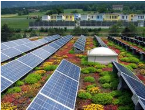
Solar panels on a green roof
