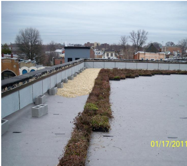
Setting the perimeter
