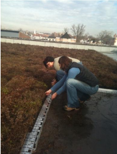
Volunteers finish installation and insert metal edging
